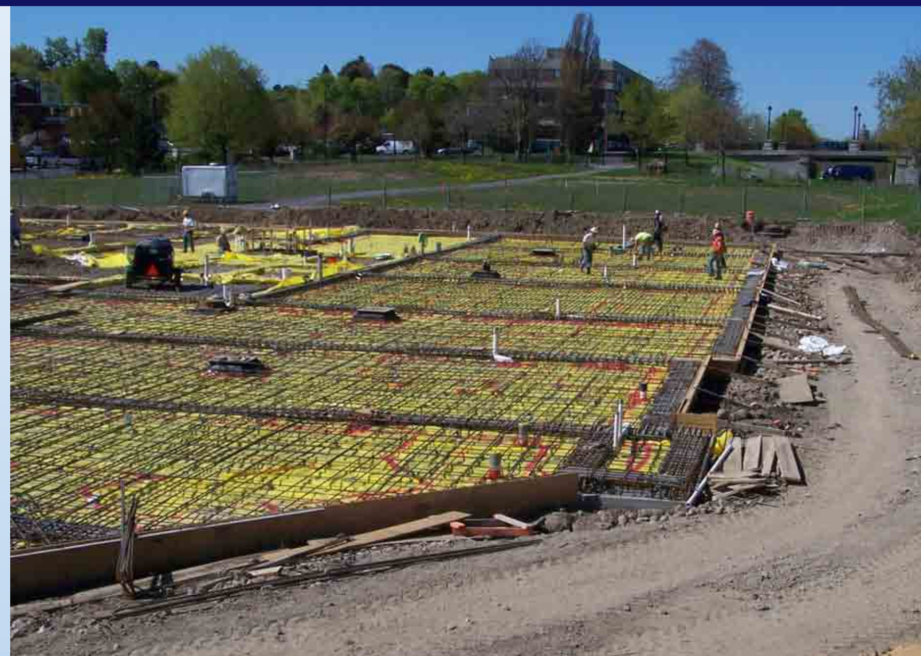
Installation of foundation system and Slab over existing pile caps.
