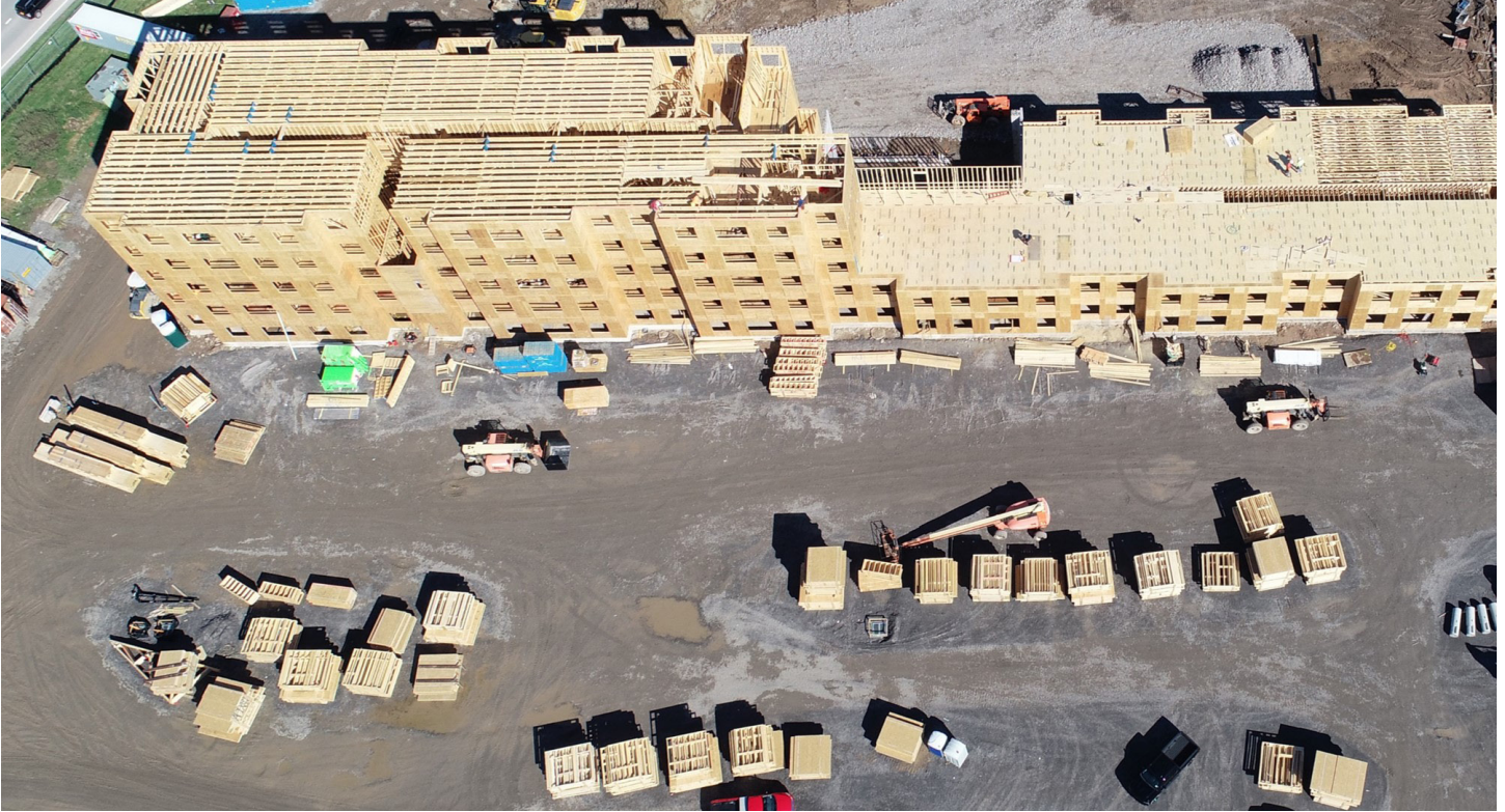
INSTALLATION OF WOOD WALL PANELS ON-SITE AT LARGE HOUSING PROJECT
